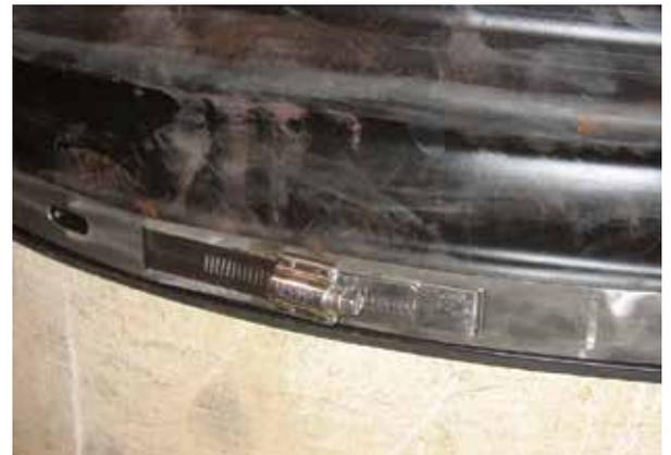
The securing band adds additional compression to the sealing fins, instantly filling any minor voids or irregularities.
