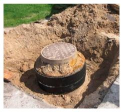
Install and center the manhole frame casting. With installation complete, backfilling and paving may proceed immediately. Take care as to not displace the rings or the frame.
