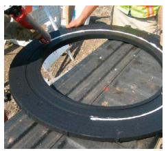
For Angle Rings, place a 1/4" bead of recommended adhesive into the groove on the underside of the Angle Ring and to the inside shoulder of the Finish Ring.
