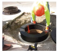
Place the Angle Ring onto the Finish Ring with the recommended adhesive facing down, making sure to align with any previously applied márks.
