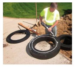
Apply a 1/4" to 1/2" bead of the recommended adhesive to the groove and to the outer glue trench of the next Grade Ring or proceed to step 10 for a Finish
